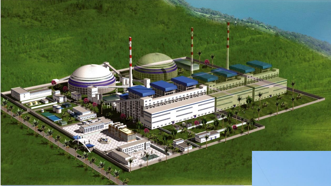
Sihanoukville 7 × 135MW coal-fired power plant aerial view
