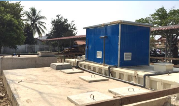
Completion of Sewage Treatment Facility
