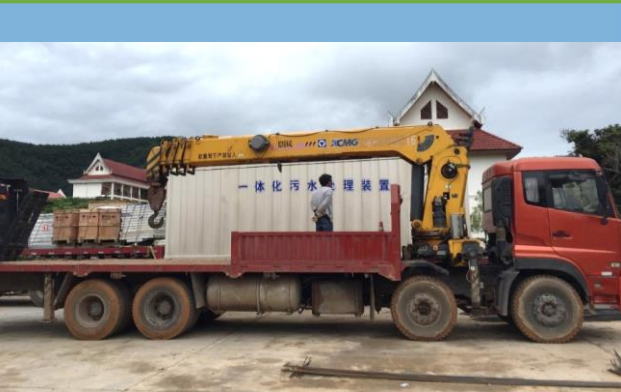
Transportation and Placement of Integrated Sewage Treatment Devices
